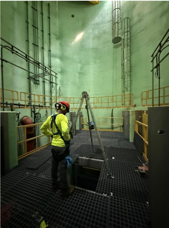
Topside grouting support in CS-12
