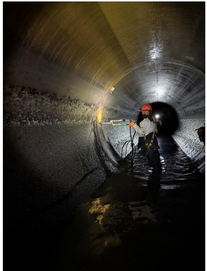
Grouting activities upstream of CS-12
