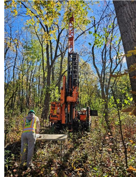
Image 1: Photo of an ATV Mounted Drill Rig during drilling activities.
