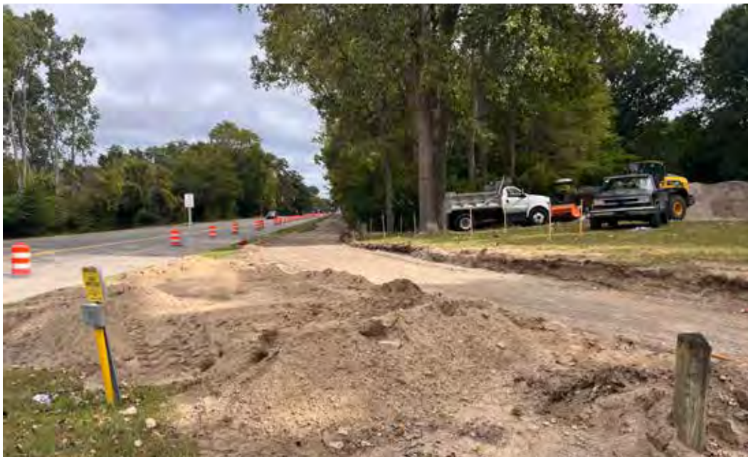
Bauervic Woods path construction.
